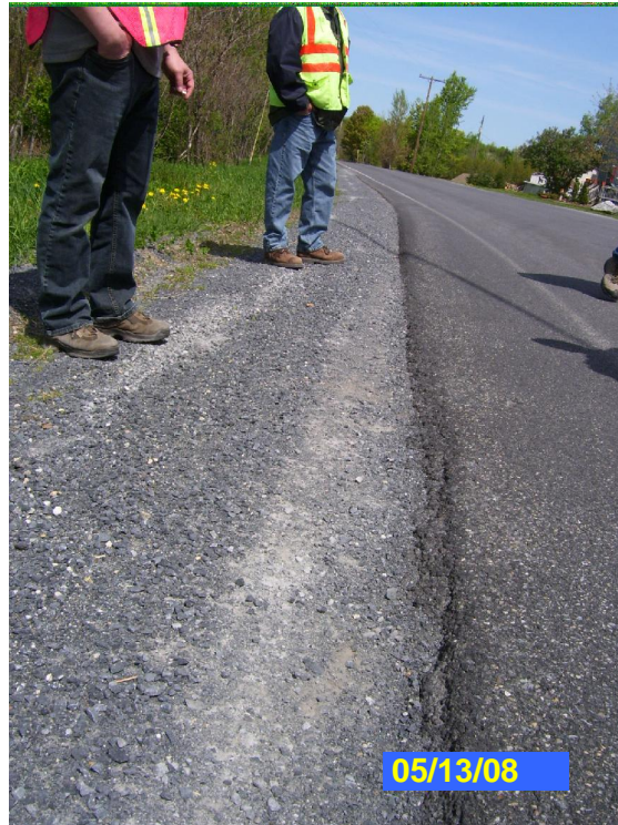
Figure 3 – Edge Drop-off
