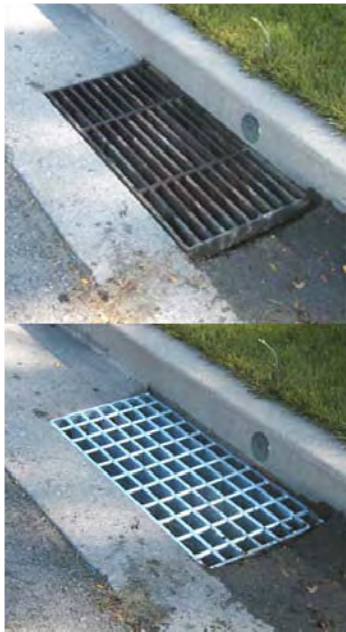
Figure 10 - Above, poor drainage grate choice; Below, bicycle-friendly grate (photos courtesy of Syrcast)
