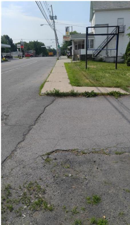
Missing ADA Ramp at commercial
