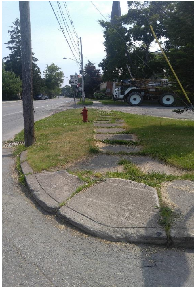
Sidewalk at southeast corner of NY Route 197 and NY Route 40: poor condition and not ADA accessible
