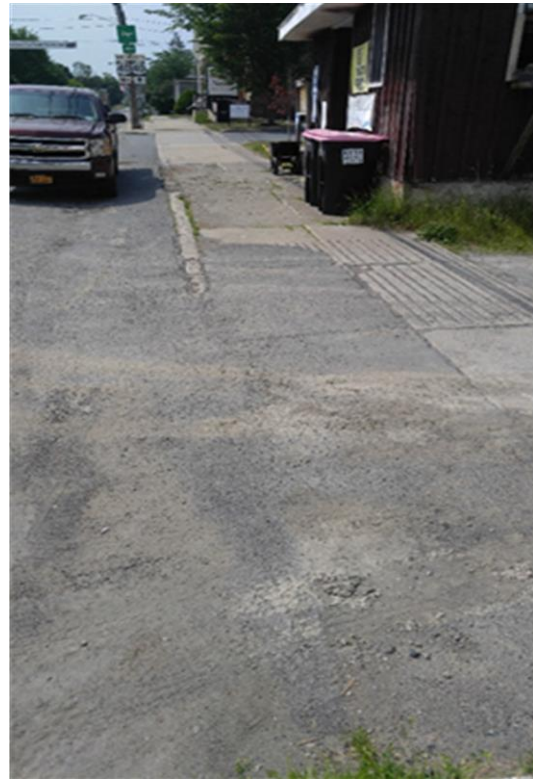
Sidewalk in front of 95 Main Street in poor condition
