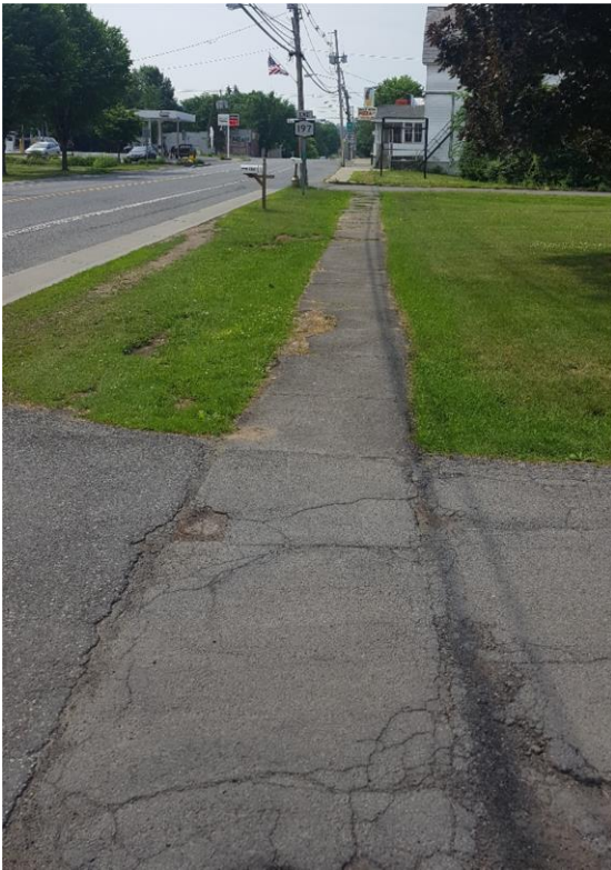
Asphalt Sidewalk Section in poor condition and narrow width
