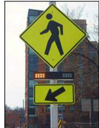
Pedestrian Crossing Signage with Rectangular Rapid Flashing Beacon (RRFB)
