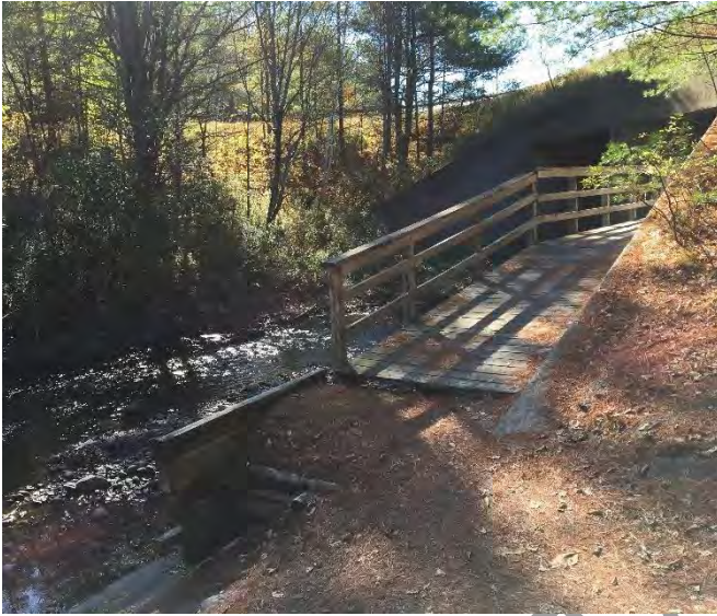
Figure 12 -- Pedestrian underpass, Carol Thomas Memorial Trail
