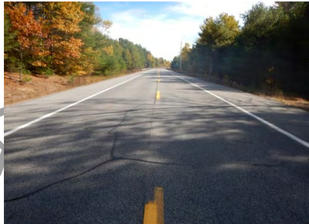
Figure 2 -- Typical Lane Configuration – Looking South from Ski Bowl Road North
