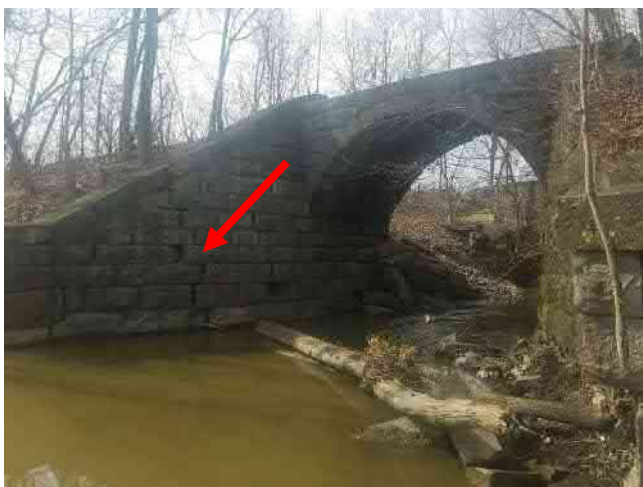
Photograph (3): General view. East Elevation. Displaced stones.
