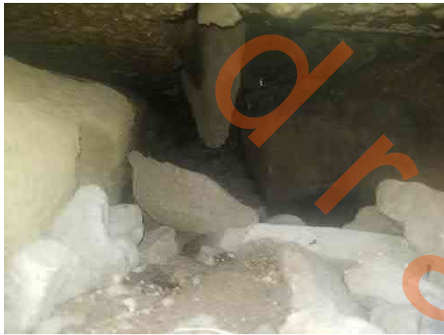
Photograph (5): Closeup view of void at southwest abutment as shown in Photograph #4.
