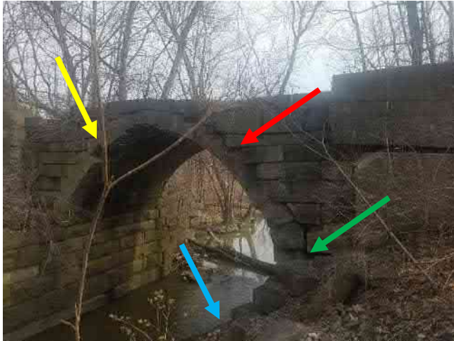
Photograph (1): General view. West Elevation (outlet). Displaced stone (red arrow), voids in abutment (green arrow) missing stone (yellow arrow).
