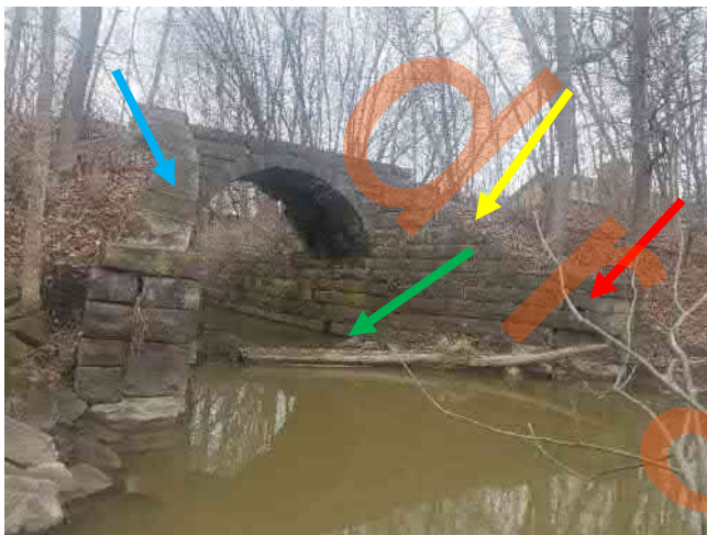
Photograph (2): General view. East Elevation (inlet). Debris restricting flow. Displaced stones (red arrow). Leaning / bulging wing wall (blue arrow). Missing cap stones (yellow arrow). Missing stone / undercut at north abutment (green arrow).
