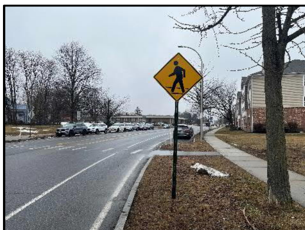
Figure 2-6: Pedestrian warning sign installed on the east approach to the Crosswalk
