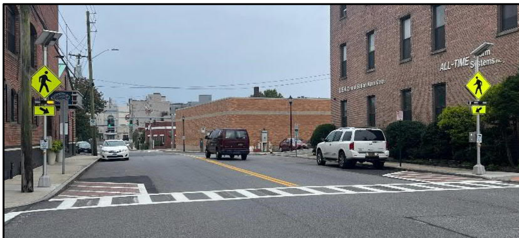
Figure 4-6: Typical RRFB Installation at an Intersection
