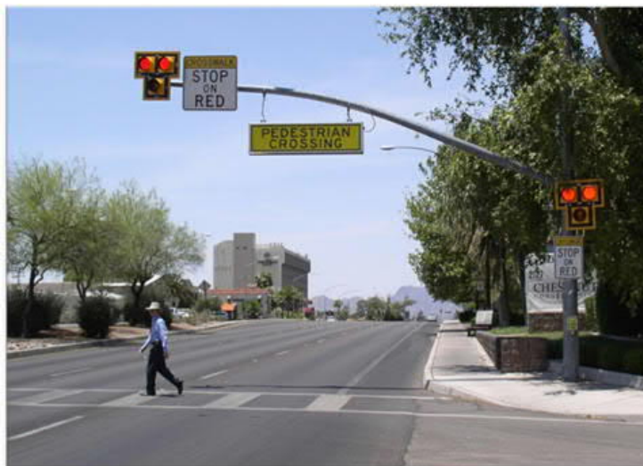
Figure 4-9: Example of a HAWK Signal in Tucson, Az.
