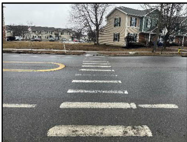
Figure 2-4: Crosswalk crossing Hudson Ave at the intersection with South St.
