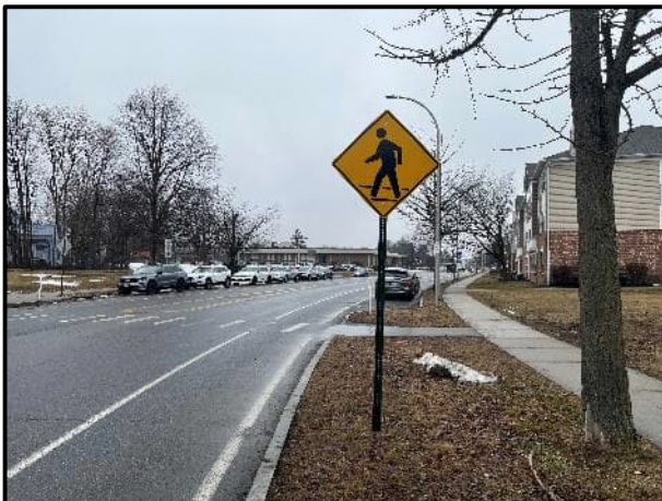
Figure 2-7: Pedestrian warning sign installed on the east approach to the Crosswalk
