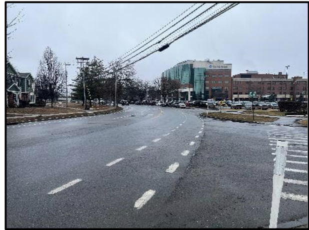
Figure 2-5: Horizontal curve on Hudson Ave looking east
