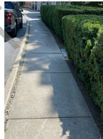
Figure III-2: 13 North St. to E. Main St.
