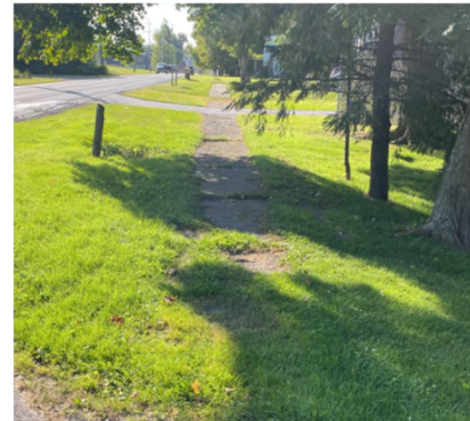
Figure III-3: Existing Sidewalk near Cove Lane intersection
