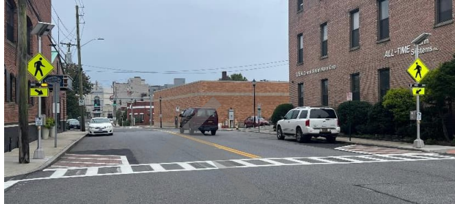
Figure III-3: RRFB Installation
