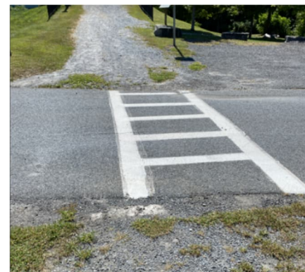
Figure II-4 – Water Street Crossing
