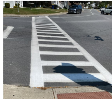
Figure II-4 Crosswalk on CR 24 and Main St.
