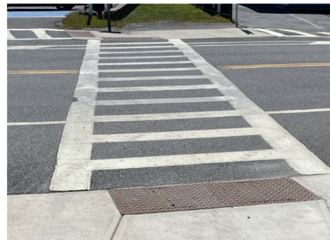
Figure III-5: Main St Crossing
