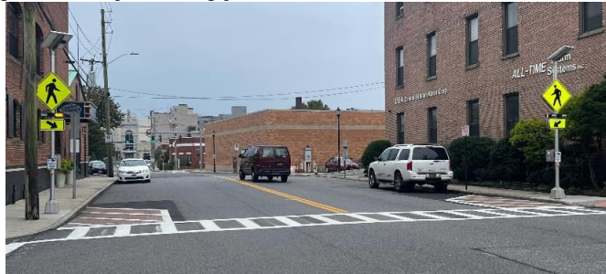
Figure III-3: RRFB Installation
