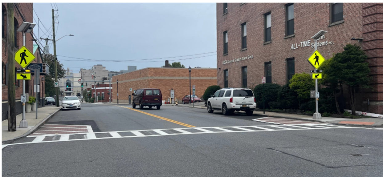
Figure 7 – RRFB's installed on a B&L Project on Abendroth Ave. in Port Chester, NY.
