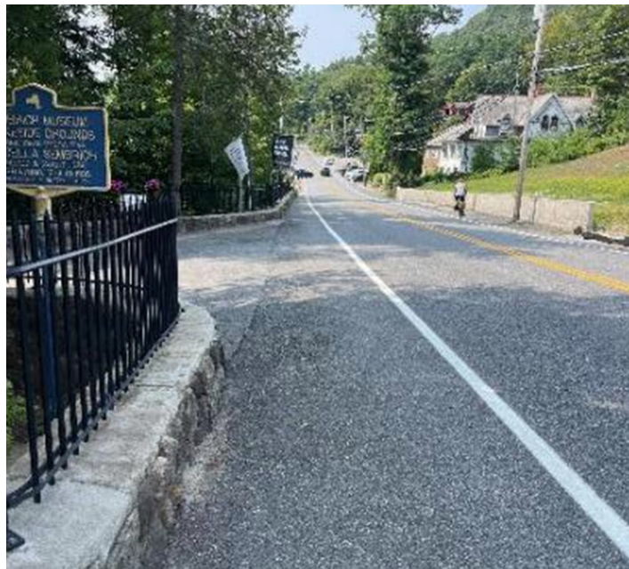
Figure 2 - Roadside conditions along the corridor, showing retaining walls on both sides of the roadway, a driveway, and utility poles on the west side.
