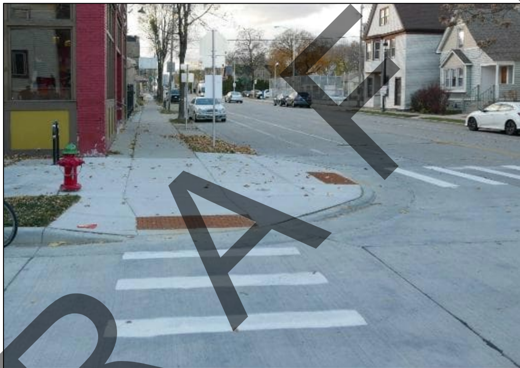
Figure 5-5 Traffic Calming Bump Outs
