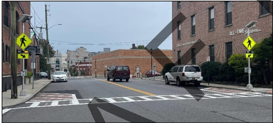
Figure 5-7: Typical RRFB Installation at an Intersection
