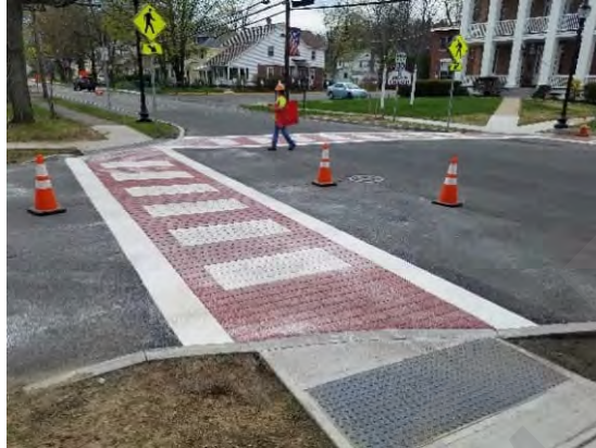
Figure 4. Imprinted Thermoplastic Crosswalks. Source: Harbour Roads and Ennis-Flint
