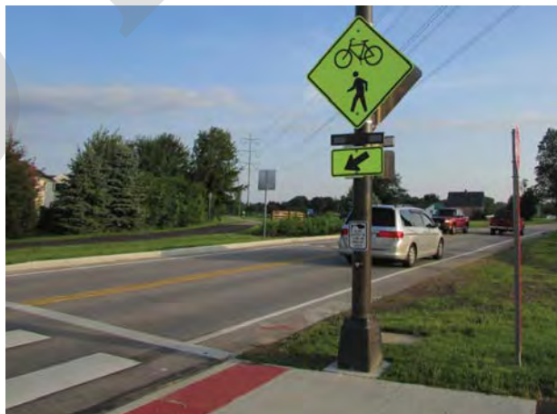
Figure 5. RRFBs Used at a Crossing. Source: FHWA
