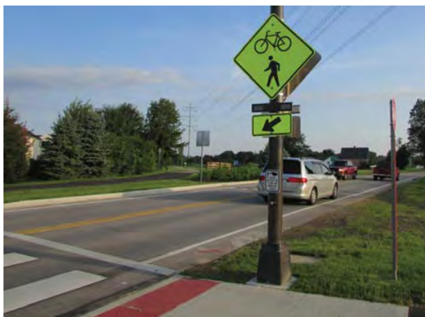
Figure 5. RRFBs Used at a Crossing. Source: FHWA
