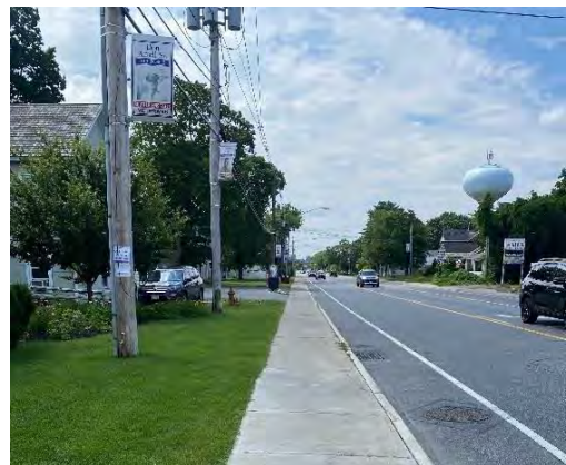
Existing Sidewalk Adjacent to Stewarts
